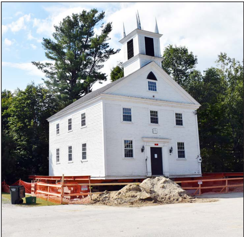
The Hebron Academy building has been raised in order to put a concrete basement under it.
