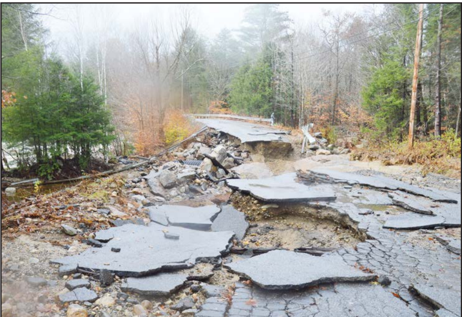
DONNA RHODES Heavy rains turned the typically peaceful Fowler River in Alexandria into a raging force of nature that clogged large drainage pipes and tore away a large section of Fowler River Road.
