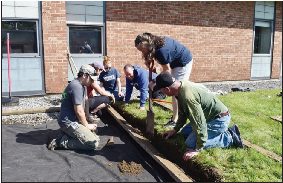
While crushed stone was being laid for the base of a hoop house-style greenhouse at Winnisquam Middle School, volunteers from both the school and Belnap Landscape Company secured the edges of the underlying landscape fabric placed over the soil.
