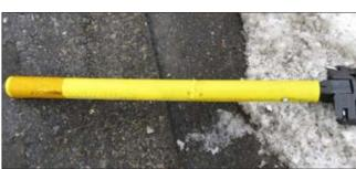
This stanchion found along Gardner Road was pulled up by a plow blade from its base which is still connected as automobiles do not sit low enough to scrap the ground.
