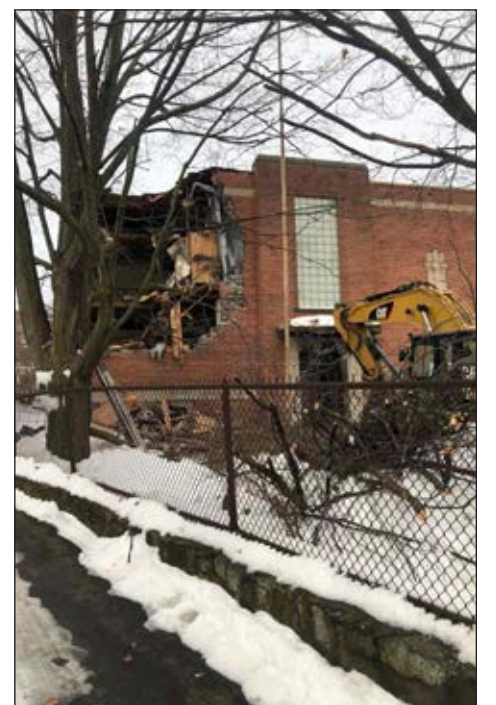
The front left side of the building is torn down first.
