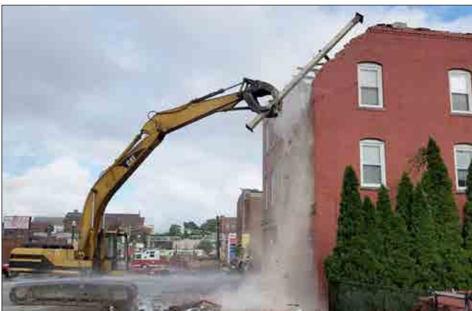
A large crane begins ripping into a building.
