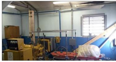
A generator bay with ceiling tiles falling apart. This also acts as a storage room for equipment in the station.
