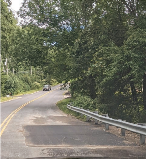
Courtesy Before and after photos of a washout on Muggett Hill Road during the Sept. 2 rainstorm and repairs made within 24-hours to make the road passable again.
