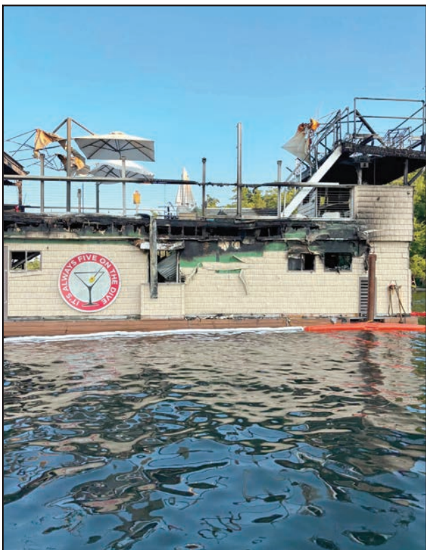
Photos posted on social media by the owners of The Dive on Winnepesaukee show the aftermath of a massive fire that destroyed the floating bar and restaurant last weekend.
