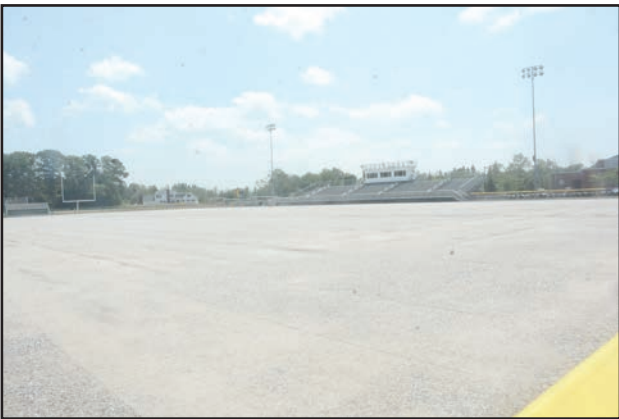
The base layer for Alumni Field was scraped off to make room for a shock pad under the new turf.
