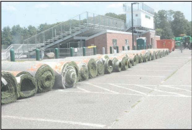
The old Alumni Field turf was rolled up and will be used to create shock pads for new turf fields like Kingswood’s.
