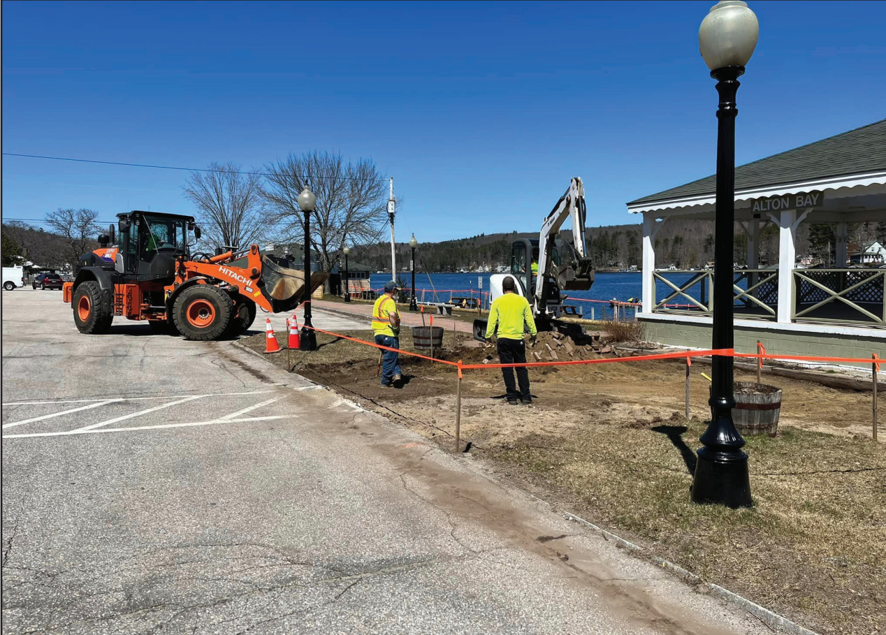
Crews tore out the old brick sidewalk and curbing before installing a new concrete sidewalk. Photo from Alton Department of Public Works' Facebook page.
