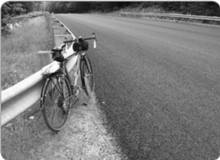
Peter Minnich New chip seal pavement, as seen near the Crawford Notch State Park pull-off. Traffic lines have yet to be applied. The vehicle travel lanes will become smoother with use, but the shoulders, where cyclists ride, will remain rough and will accumulate loose aggregate.
