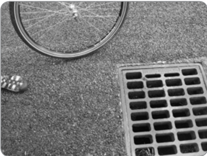
Peter Minnich Close-up of the chip seal surface with three-eighths inch aggregate. The 37c tire in the photo handles the rough surface adequately.
