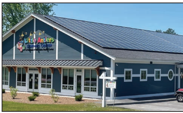
Solar panels at Mid-State Health Center's Little Antlers Learning Center, Plymouth. COURTESY
