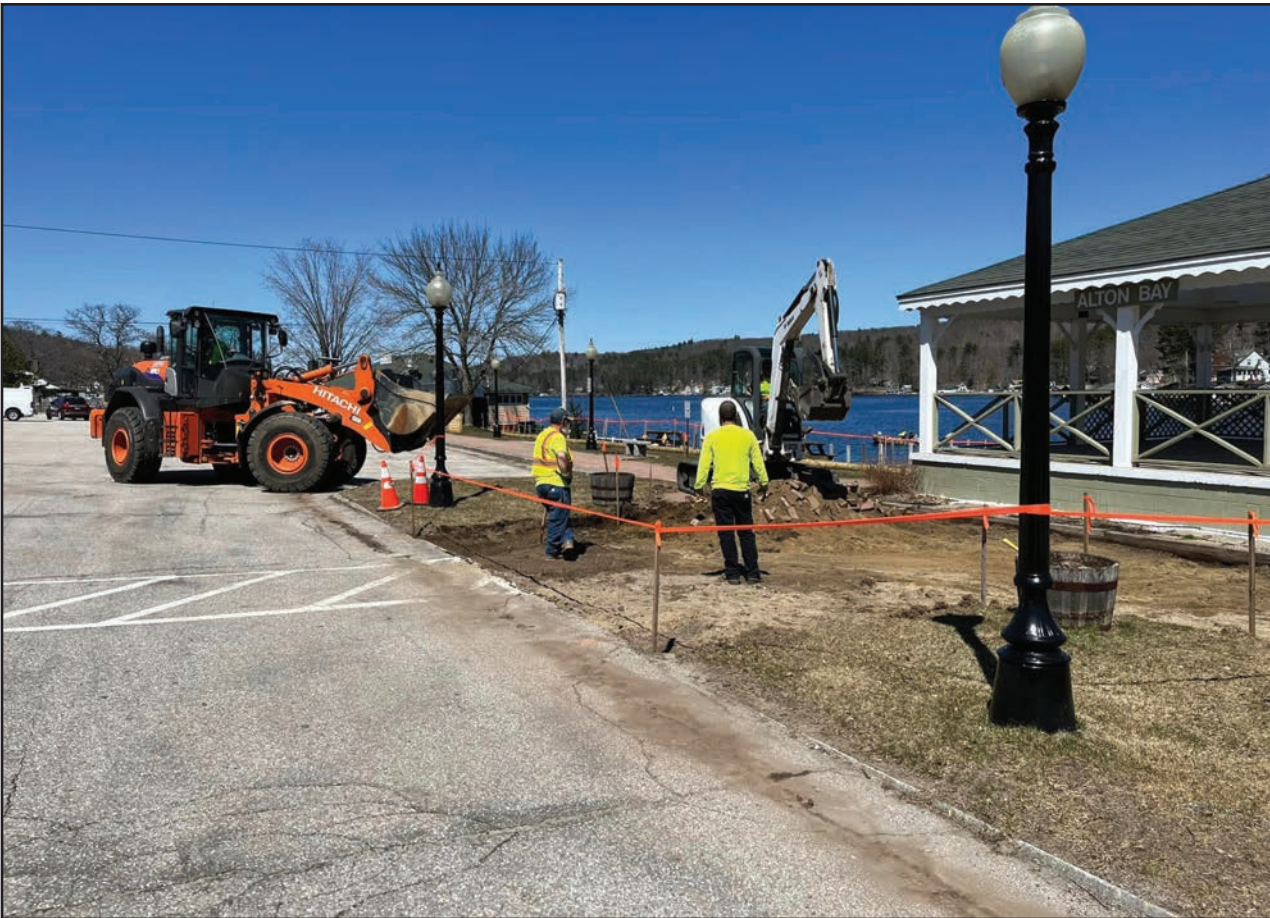
Crews tore out the old brick sidewalk and curbing before installing a new concrete sidewalk. Photo from Alton Department of Public Works' Facebook page.
