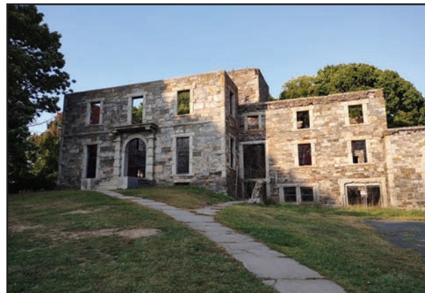
The remains of the Goddard Mansion at Fort Williams. The exterior remains, but the interior has collapsed and is fenced off.
