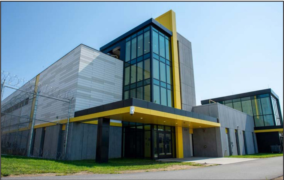
WCSO Intake/Medical Build, built in 2021, where the Safekeep program is facilitated out of.
