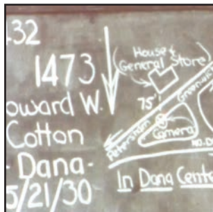
One of the engineers' photo ID signs shows where the Howard Cotton home and store once was in Dana.
