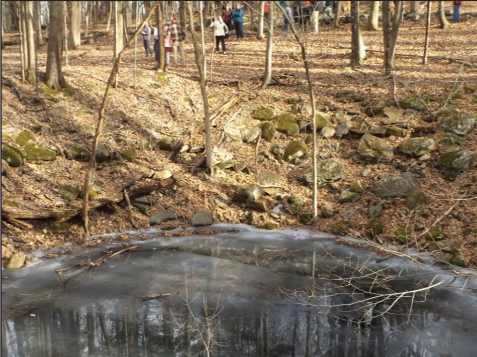
The tour explores the hilltop cistern, which is actually a little off its namesake trail. Its age is somewhat uncertain – probably early 1900s – but it was built to hold water for firefighting, with gravity providing enough pressure to serve several mills downhill along the river.
