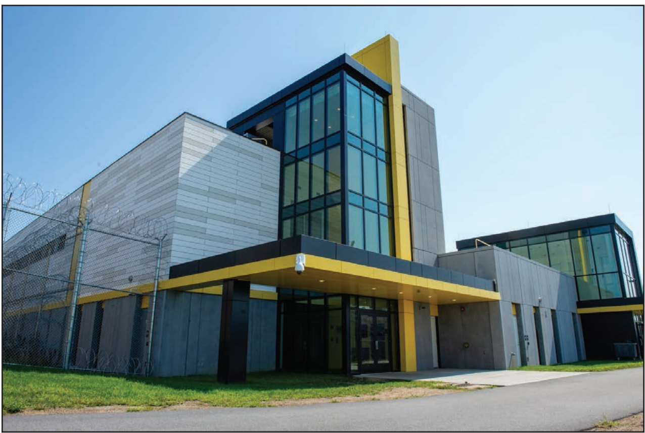
WCSO Intake/Medical Build, built in 2021, where the Safekeep program is facilitated out of.
