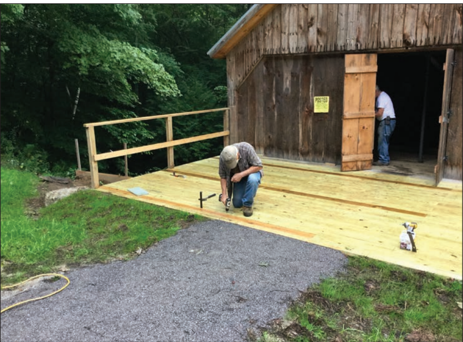
Andy Quigley screwing down decking planks.
